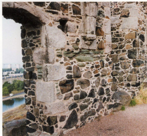
Chapel: stones mostly basalt with some ash (greenish); and pale freestone sandstone for carved work
